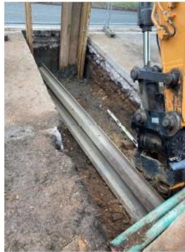
Photo of excavator arm used for task
