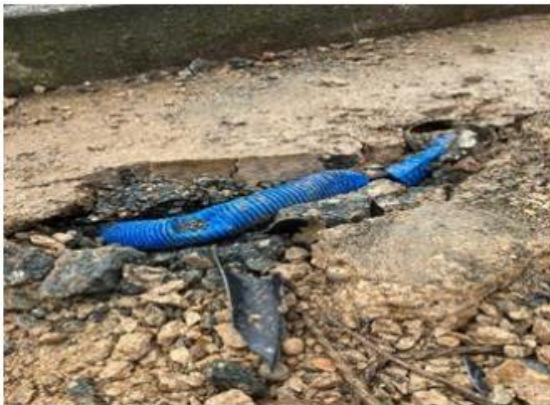
Route of cable through slab
